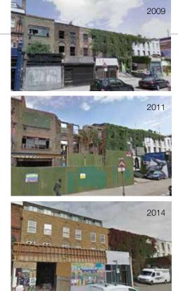
transpired that the removal of ground floor walls to achieve open plan retail space made it technically impossible to support the Georgian brickwork above.
