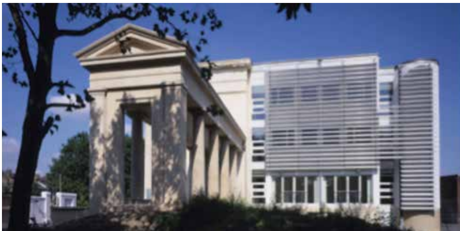
Portico Extension by Brady Mallalieu Architects, c2006
