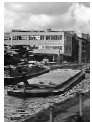
Above: River Lea and the Lesney factory in the background.
