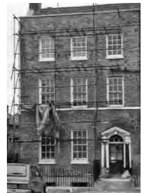
Above: Georgian terrace being restored, Stoke Newington Church Street.
