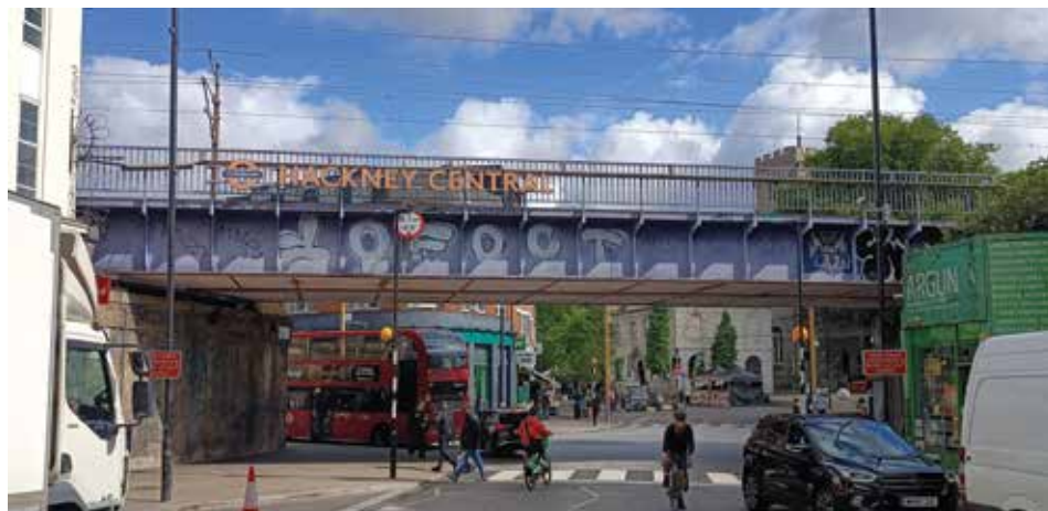
10FOOT tag on the Hackney Central railway bridge
