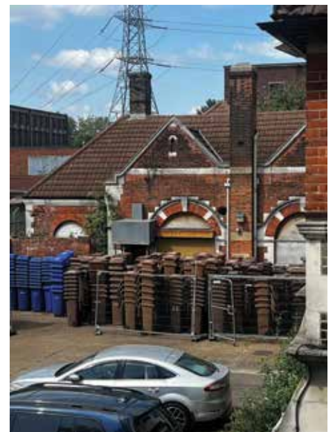
The Disinfecting Station seen behind piles of council bins April 2026 - picture Rob Briggs
